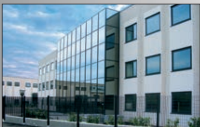
NEW PRODUCTION PLANT A.M.T S.R.L. - CASELLE T.SE - TORINO - ITALY
