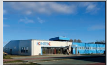
MAIN PRODUCTION PLANT KINTEK TOOLING KFT - BEKESCSABA - HUNGARY
