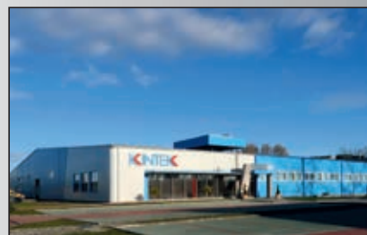
MAIN PRODUCTION PLANT KINTEK TOOLING KFT - BEKESCSABA - HUNGARY
